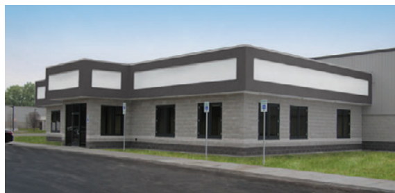
Boyne City Facility
