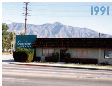
Original site, Glendale, California
