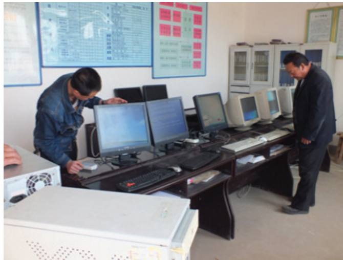
Testing the computers after installation.
