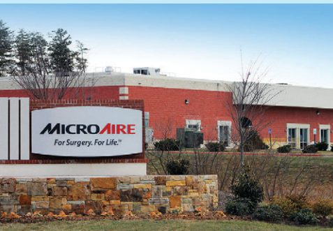
Manufacturing facility and warehouse, Charlottesville, Virginia
